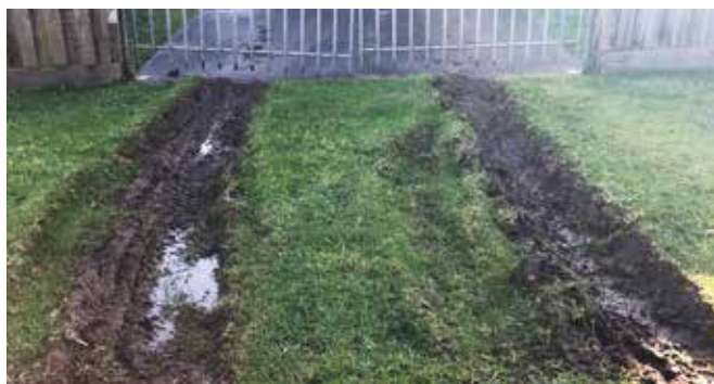
Saturated ground surface on a Gilmore Street crossover
